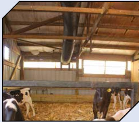
An intake fan and conduit in the rafters delivers consistent fresh air to the Hesses’ calf barn.
