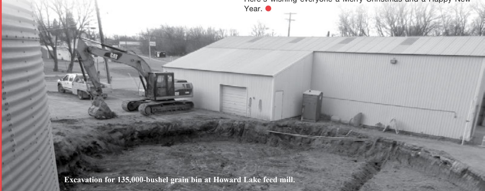
Excavation for 135,000-bushel grain bin at Howard Lake feed mill.
